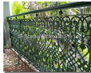
Cast Iron Balconies
